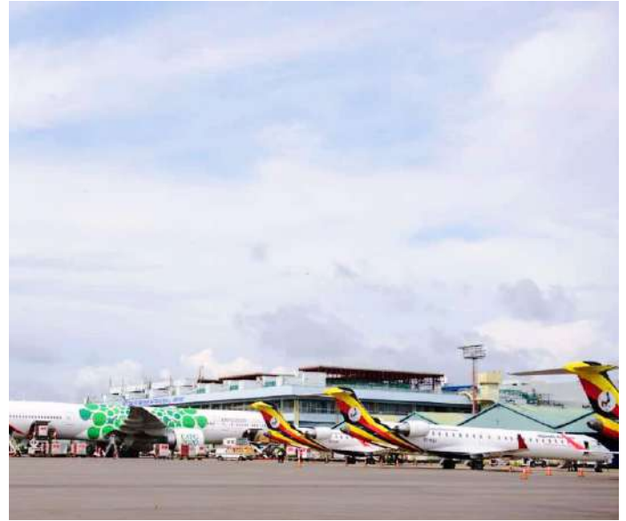
Aircraft parked at the expanded aircraft parking apron at Entebbe International Airport
