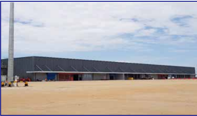
Apron side of the Cargo village building and New Apron
