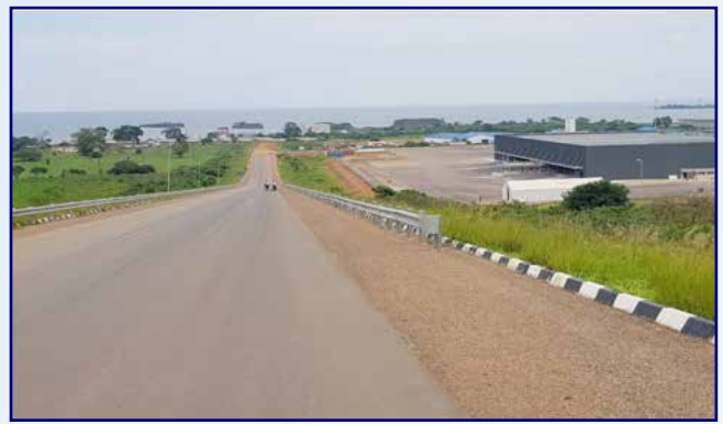
Access road to cargo village
