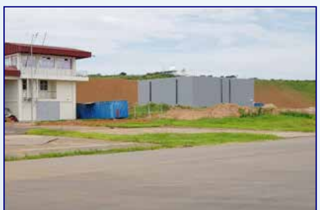
New fire station water tank
