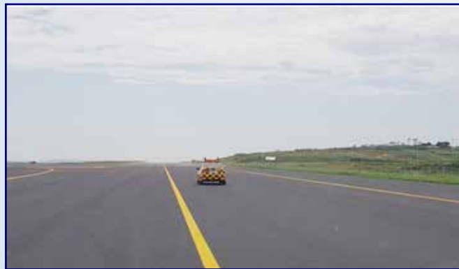
Resurfacing of the runway completed
