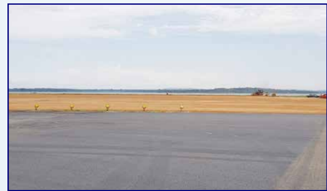
Runway extension being completed
